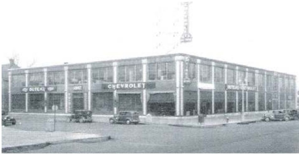
Integration of Old and New Award: Duteau Building rehabilitation
